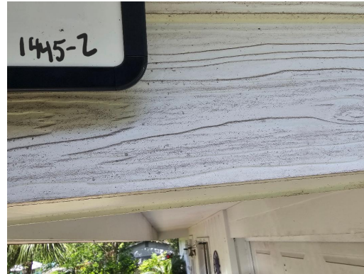
1445-2 Fibrous Siding Typical Exterior Walls
